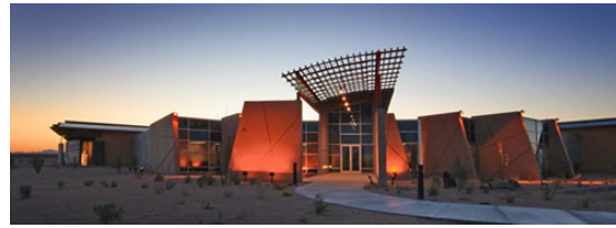
Butler Water Reclamation Facility
